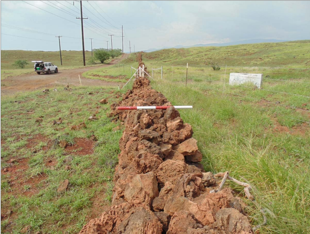
Figure 35. SIHP Site 9012, top surface of wall, view to the north.
