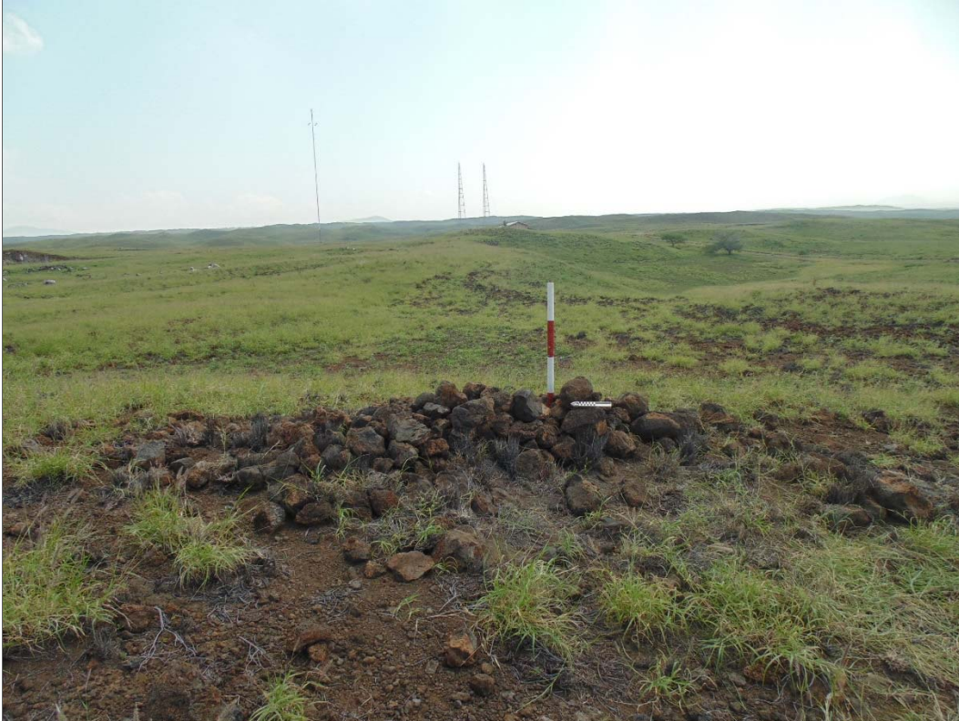
Figure 45. SIHP Site 30109 Feature G, collapsed wall segment, view to the east.
