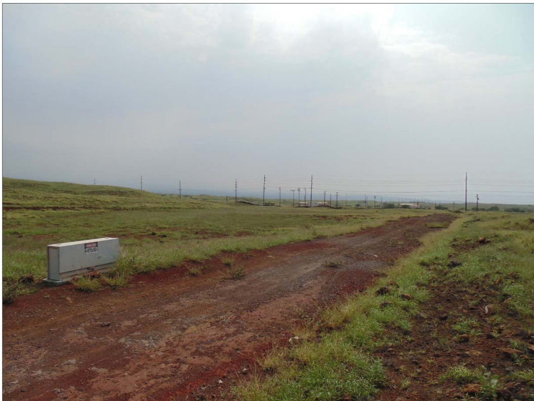
Figure 8. Lālāmilo survey area, electrical along the southern edge of the existing road, view to the southwest.
